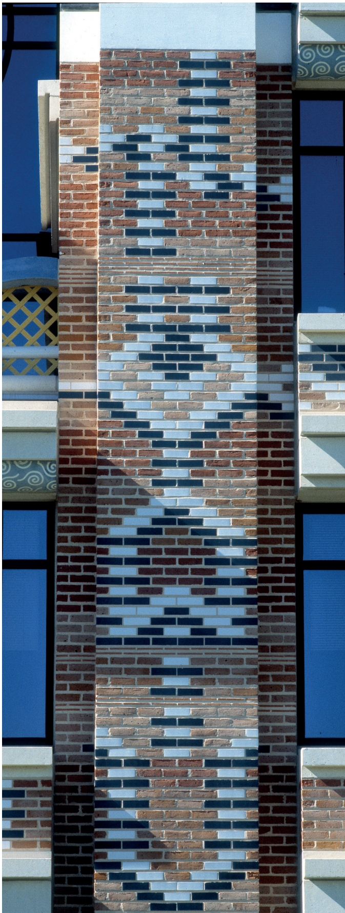
The four states of matter signed in 'Vedic' guise are inlaid in dark blue (black was too violent) and white glazed bricks. This detail shows the striations of the four different colours of bricks from St. Joe's brickworks in New Orleans. Note the 'coursing tiles' that also striate the flanks of the Mountain of the Genius Loci.
